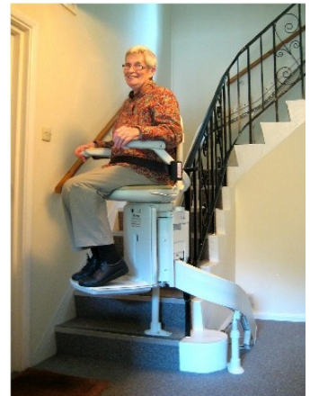
The Stairlift in Morley House
