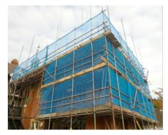
Like much of the rest of the building, the main chapel has disappeared beneath a maze of scaffolding and blue protective netting (*left*) and is soon to be covered with a protective 'tin roof'. This is because the project involves re-roofing the whole of the central block, including the chapel and kitchens, as well as the eastern section of the main College building. Our 'green' credentials will also be enhanced as huge amounts of insulation and many new windows are installed.
